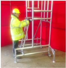
5) CLIP UPPER BRACE OF LADDER ABOVE RINGS ON VERTICALS WITH ASSEMBLED HOOKS ON TOP
