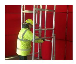
1) OPEN FRAME AND LOCK MECHANISM
