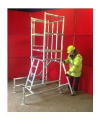
6) DEPLOY STABILISERS IN CORRECT POSITION
